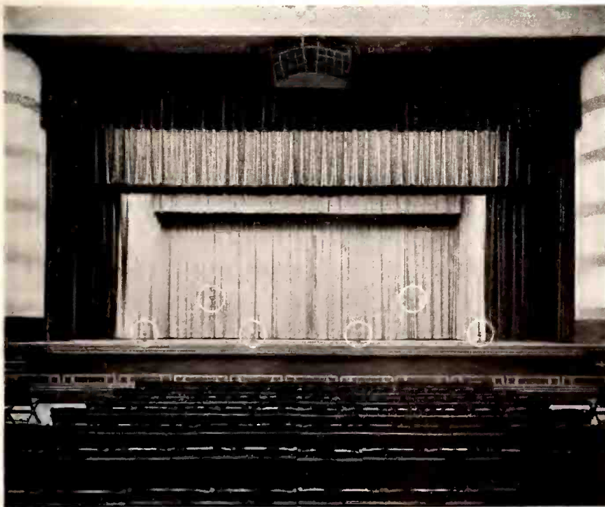
Microphone and speaker layout on stage of Kansas Civic auditorium. Foot-light mikes (in lower circles) operate at full gain. Frequencies below 250 cycles are cut off and only wide-angle HF horns are used.
